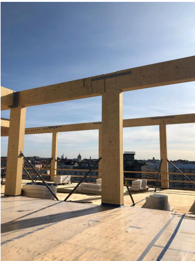
Figure 44: Left: Bolted connection for LVL G columns on construction site (Wood city project, Finland); Right: Screwed connection for LVL G trusses in delivery (Ydalir project, Norway)
